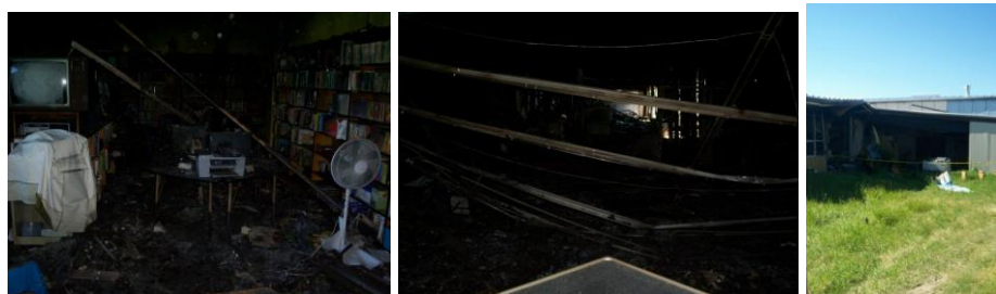
Figure 12. Aftermath of the 2008 fire. Photographs courtesy Adam Peterson.
